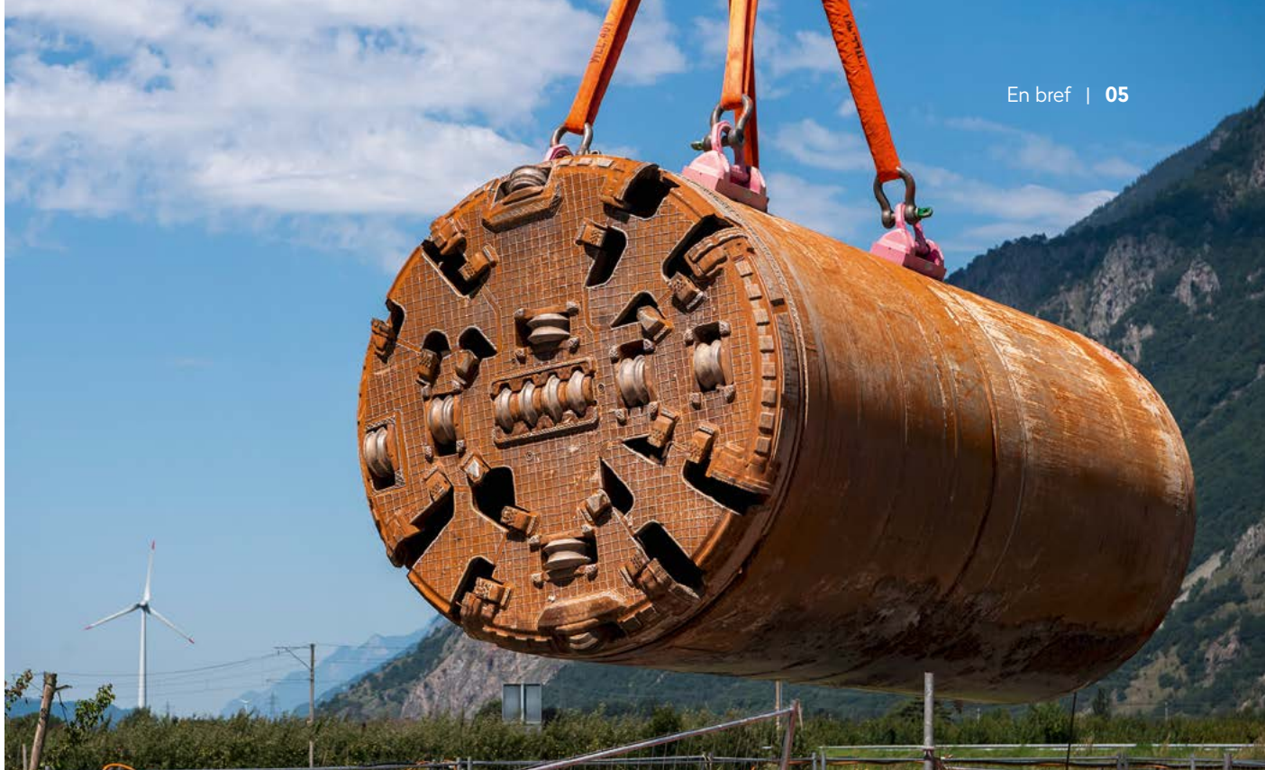
↑ Mini-tunnelier «Giorgia» – Martigny, 12.08.2021 – © KEYSTONE, Jean-Christophe Bott
